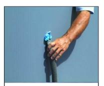
Tape up skimmer hole with cardboard and put the vacuum hose through the return hole in the wall so the hose is between the pool wall and the liner.
