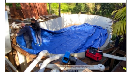
Put the liner wall up over the pool wall and hold in place with the plastic coping strips. Adjust the overlap to remove all wrinkles.
